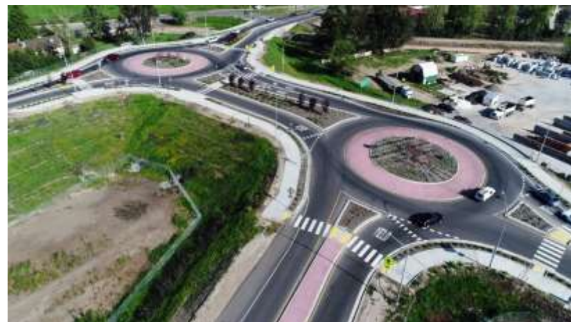
SR-198 and Farmersville Blvd Roundabouts (Farmersville, CA)
